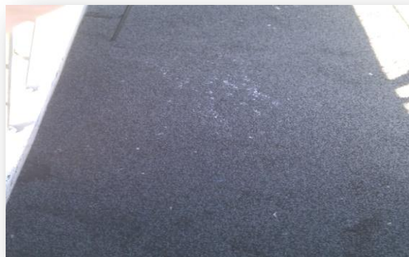
曝气池填料导到了缺氧池
